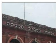
RAILING (FOR TOE WALL AND PARAPET)
