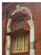
CHHAJJAS (FOR SHADING DEVICE)
